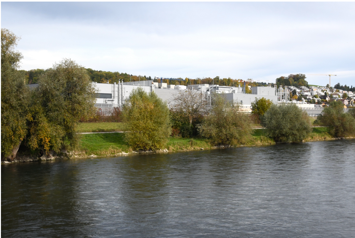
Figure 21: Data Center by a River
