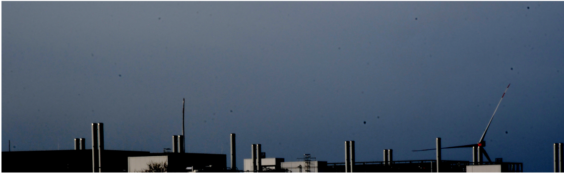
Figure 20: Flues of a Data Center in Brandenburg
