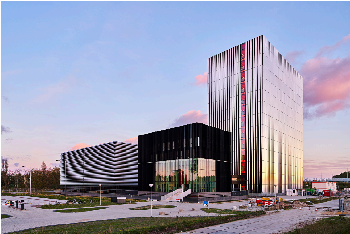
Figure 2: Equinix AM4 Data Center, Amsterdam
