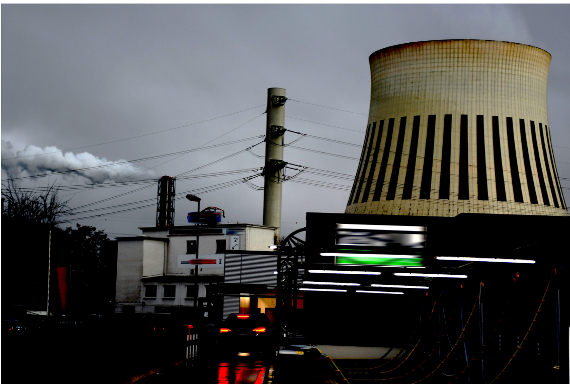
Figure 11: Combined Heat and Power Plant
