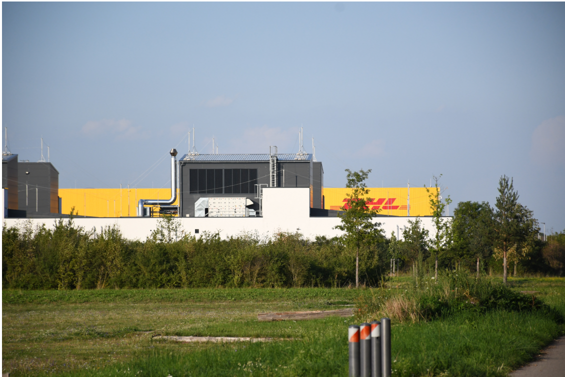
Figure 6: Parcel Center Behind Data Center
