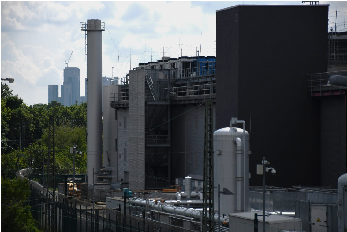
Figure 7: Data Center in Industrial District with City Skyline in the Background
