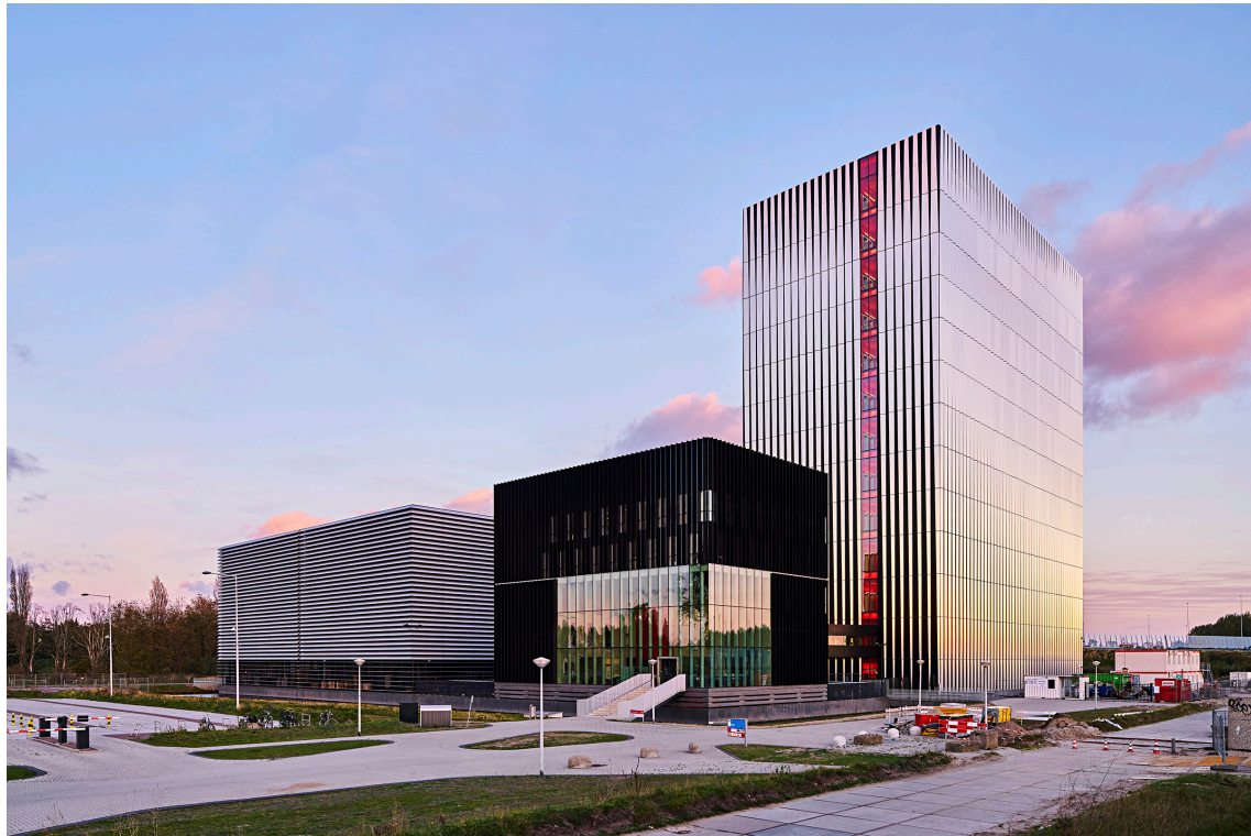
Figure 2: Equinix AM4 Data Center, Amsterdam
