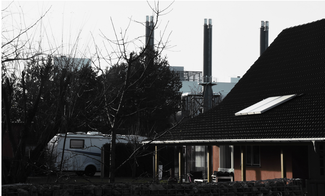
Figure 8: Data Center in a Rural Village
