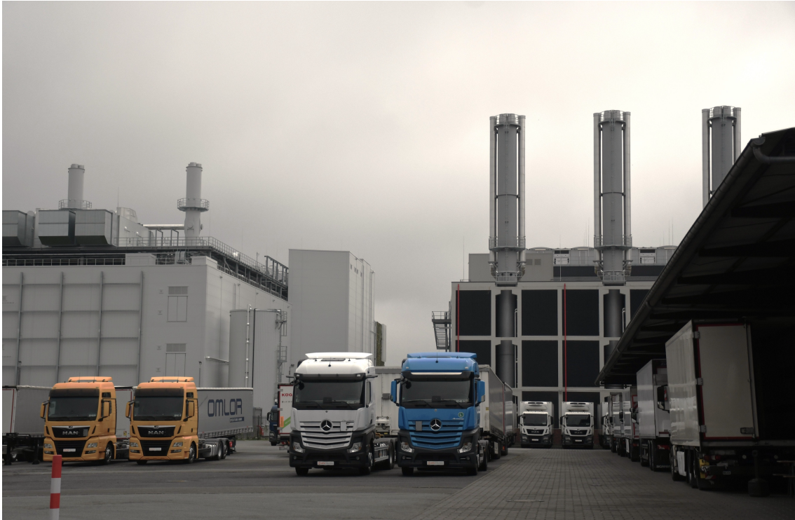
Figure 5: Logistical Services behind a Data Center
